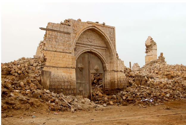
Figure 2. Deterioration of Suakin's historic coral block buildings
